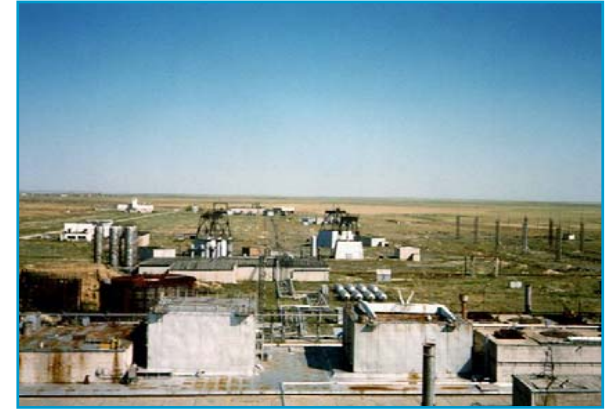
“Baikal-1” Reactor Complex
